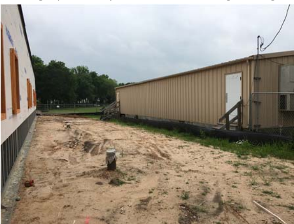
Photograph 14. Oyster Creek Showing Fire Egress from Portable Units
