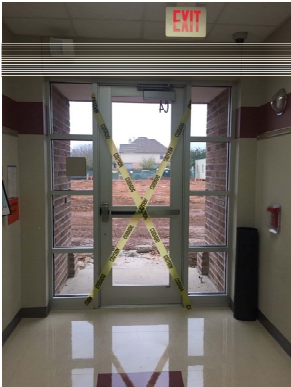
Photograph 12. Cornerstone Elementary School Emergency Exit
