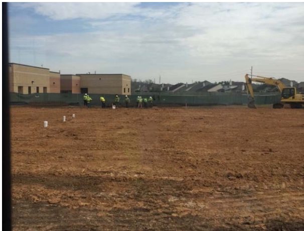
Photograph 6. Schiff Elementary Construction Site Fencing, January 2017
