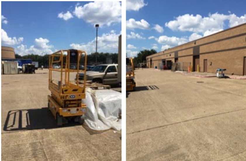
Photographs 1 and 2. Clements High School Job Site
