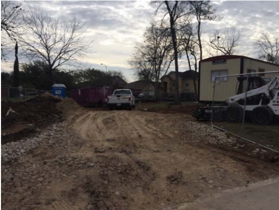
Photograph 13. Oyster Creek Construction Entrance
