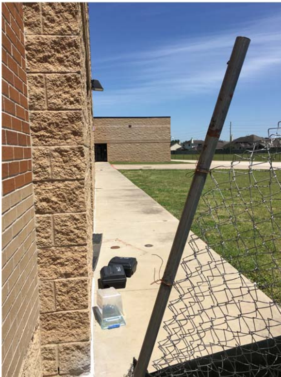
Photograph 10. Schiff Elementary Construction Fence not attached to the school, April 2017
