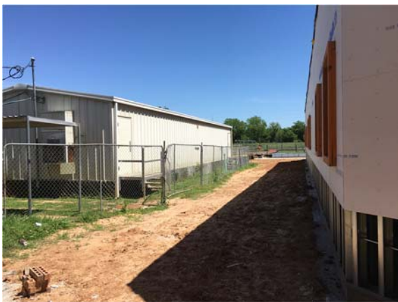
Photograph 19. Sienna Crossing Fence away from Portables Fire Exit
