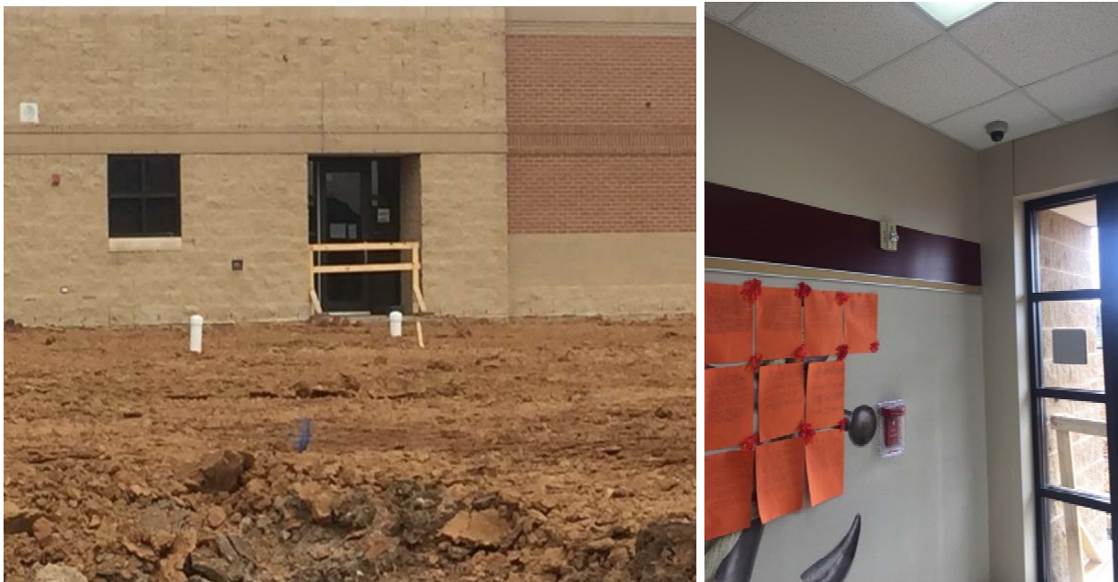
Photographs 8 and 9. Schiff Elementary Emergency Exit, January 2017
