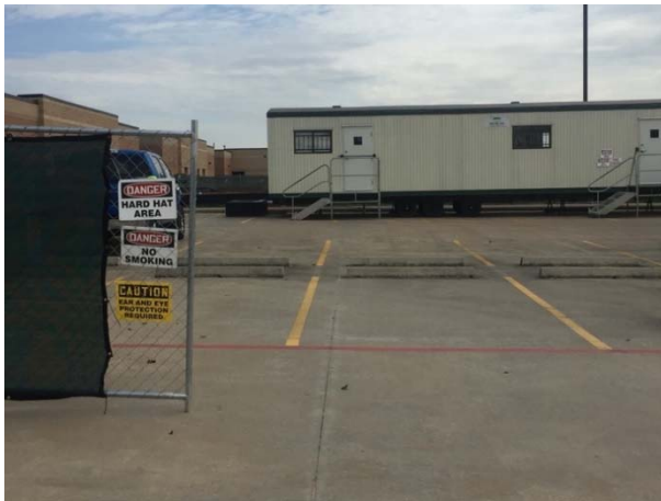
Photograph 7. Schiff Elementary Construction Site Entrance, January 2017
