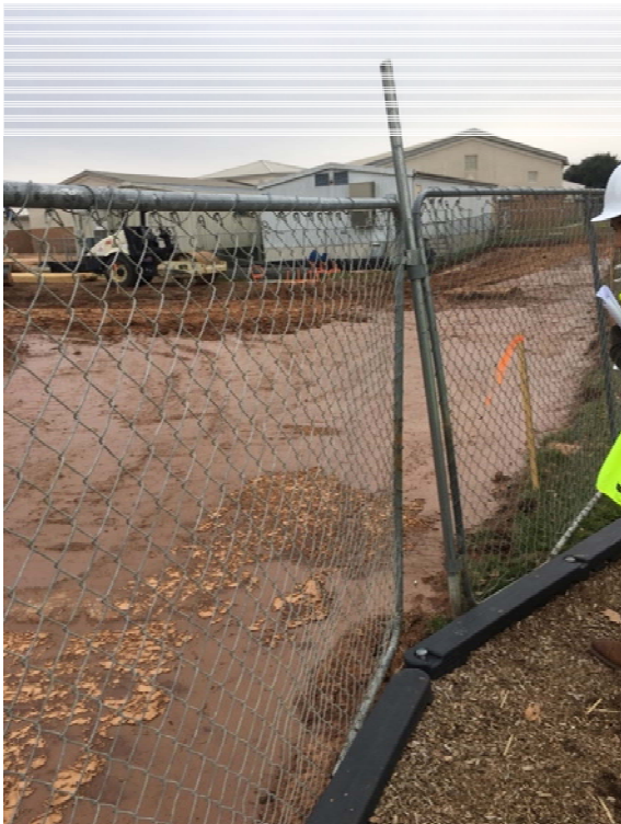
Photograph 17. Sienna Crossing Construction Fence
